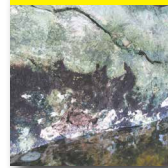
Before: Seawall Facing In Need of Repair
