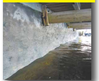
After: Seawall Face Repaired
