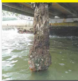
Before: Borer Worm Damage
