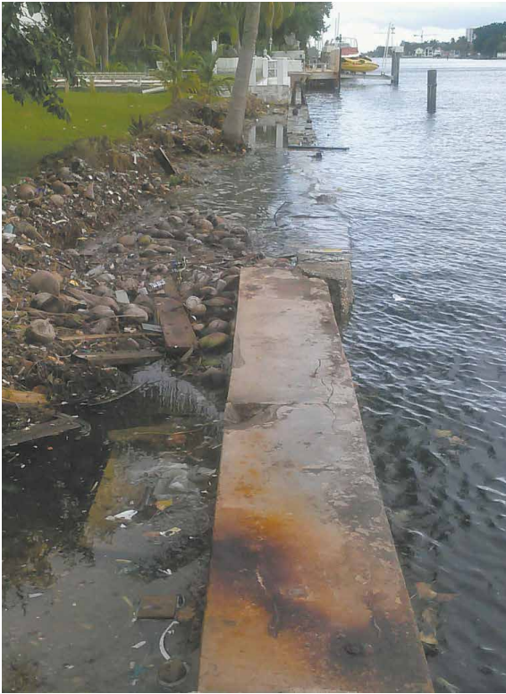
Before: Borer Worm Damage
