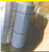
After: Pile Restoration
